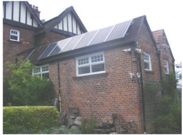
PHOTO 2 Southern Elevation of Extension
