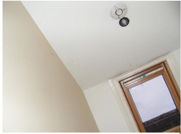
PHOTO 16 Underside of Western roof
