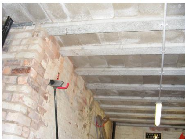
PHOTO 21 Underside of Main Cellar Roof
