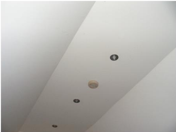
PHOTO 17 Underside of Extension Roof
