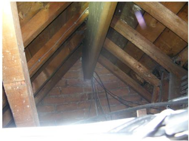
PHOTO 14 Underside of Southern Roof
