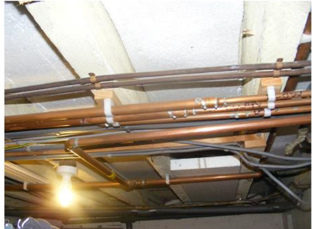
PHOTO 18 Underside of Cellar Roof
