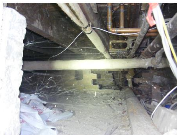
PHOTO 19 Underside of Utilities Tunnel
