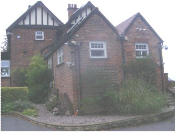
PHOTO 1 Eastern Elevation of House
