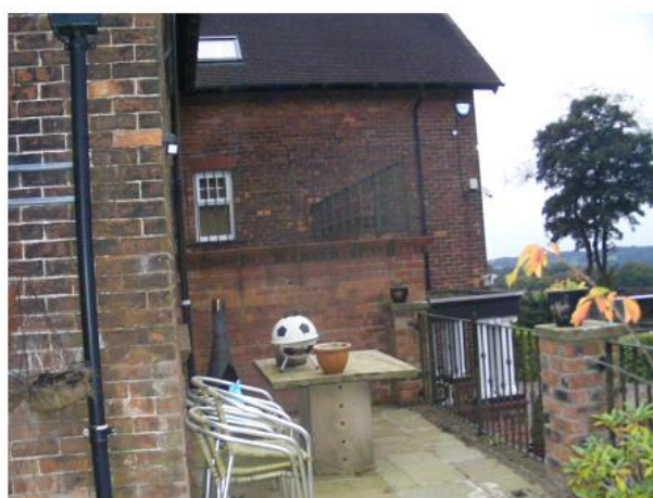
PHOTO 20 Eastern View of Balcony
