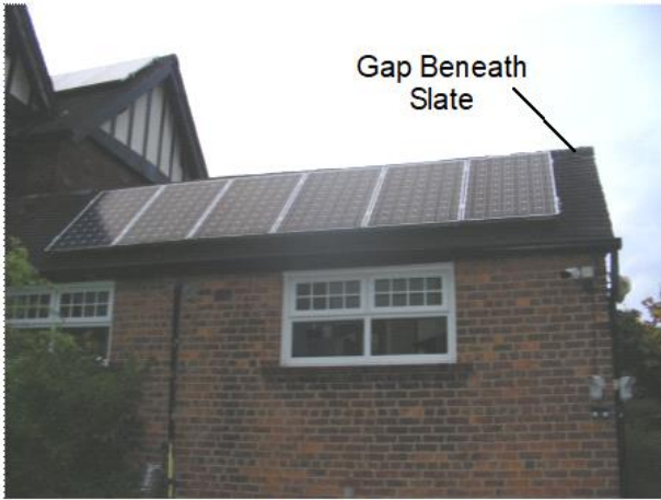
PHOTO 13 Southern Elevation of Extension
