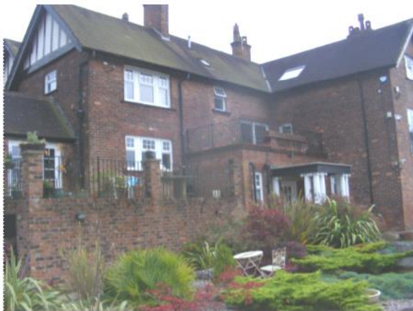
PHOTO 11 Part Northern Elevation
