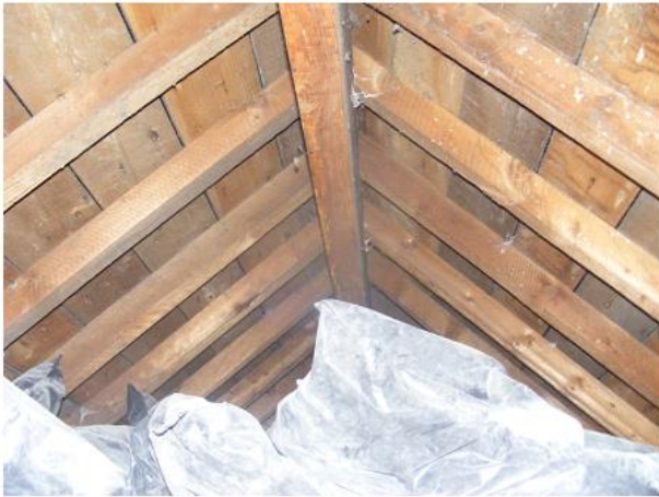
PHOTO 15 Underside of Northern Roof
