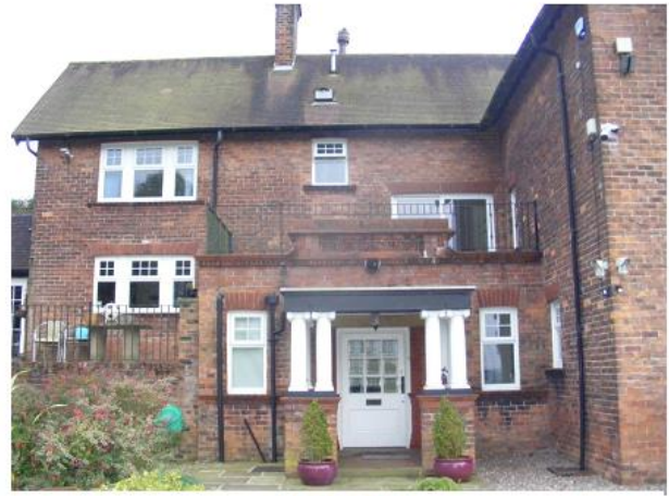
PHOTO 10 Northern Elevation of Entrance
