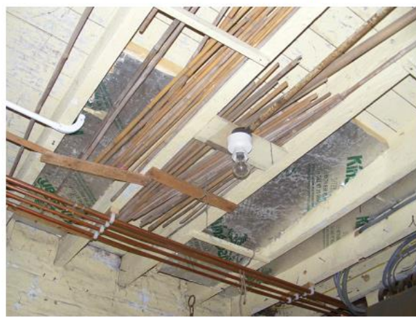
PHOTO 22 Underside of Crawspace roof
